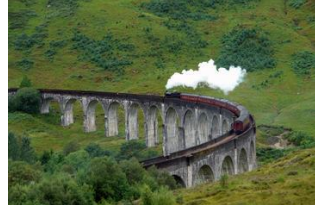
Viaduct at Glenfinnan
